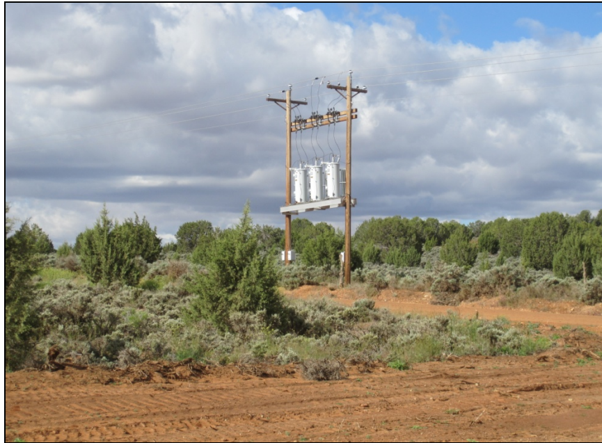
Figure 3-13. Transformer Substation on Old Landfill Road adjacent to Proposed Pilot Plant Site
