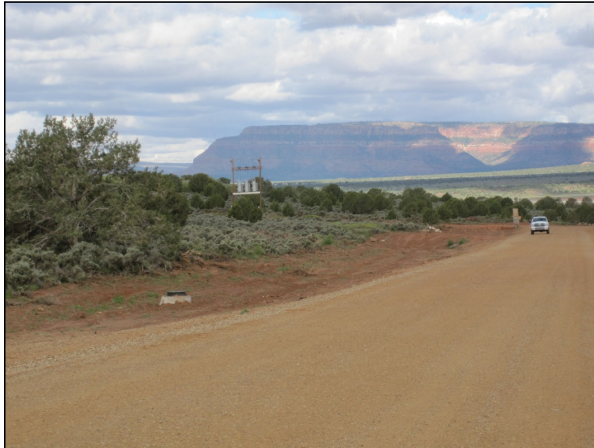
Figure 3-12. Sanitary Sewer on Kaneplex Road at Proposed Pilot Plant Site (recently installed to serve Public Safety Facility)
